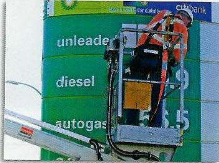
Maintenance work for BP Australia.
